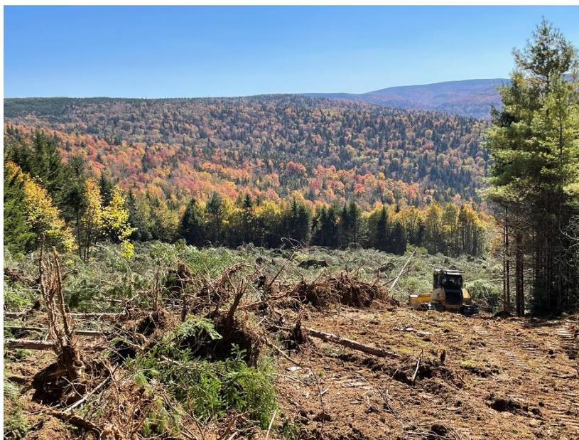
*Amid fall colors, heavy machinery push stunted, non-native conifers out of the way before decompacting the soil at Mower 23/Fish Hatchery in preparation from spring tree planting.
